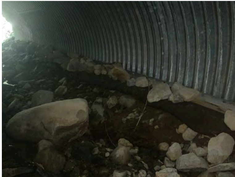
Right Bank Abutment when facing downstream
