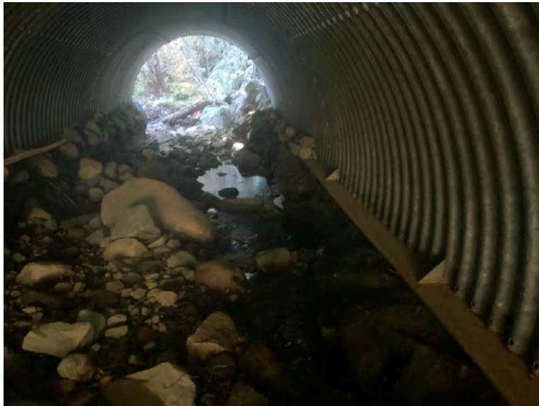
Right Bank Abutment when facing downstream
