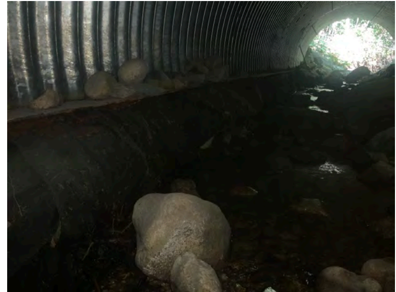
Left Bank Abutment when facing downstream
