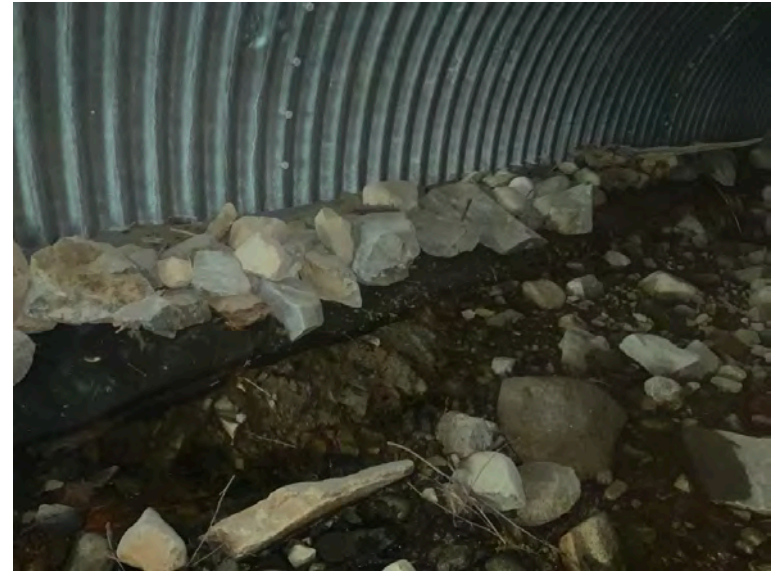
Left Bank Abutment when facing downstream
